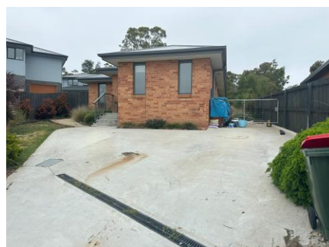
Parking area in front of existing dwelling
