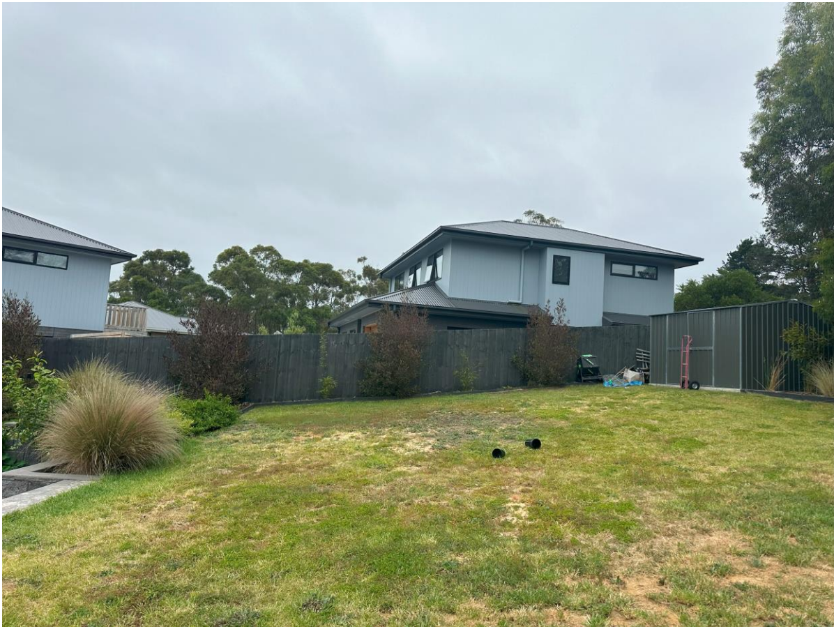
1 - View to the North
