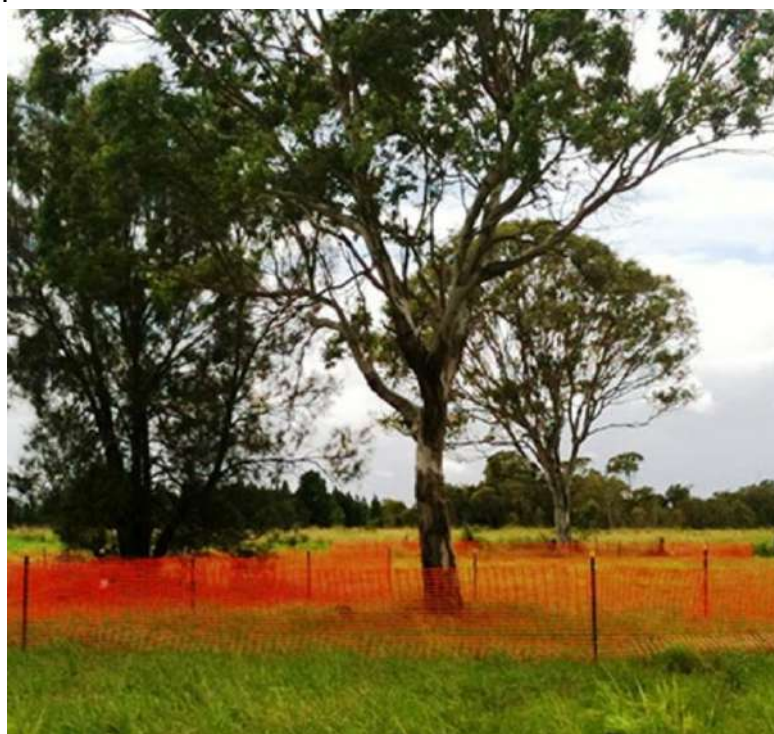
Figure 4- Tree Protection Fencing constructed with barrier mesh.
