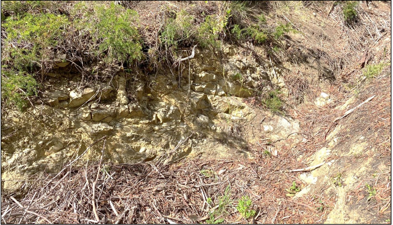
Figure 3: Shallow cutting into the hard weathered dolerite bedrock. Cutting forms the roadside stormwater drain at the north of the site.
