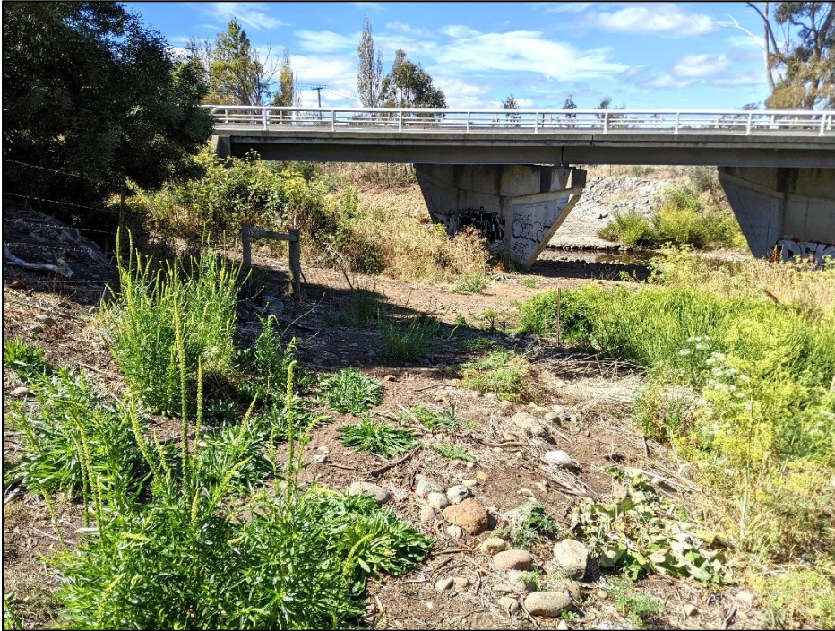
Photo 5. Disturbed area with numerous weed species in riparian zone near Channel Highway. Proposed trail route in centre of photograph, continuing under the highway bridge to Margate trailhead.
