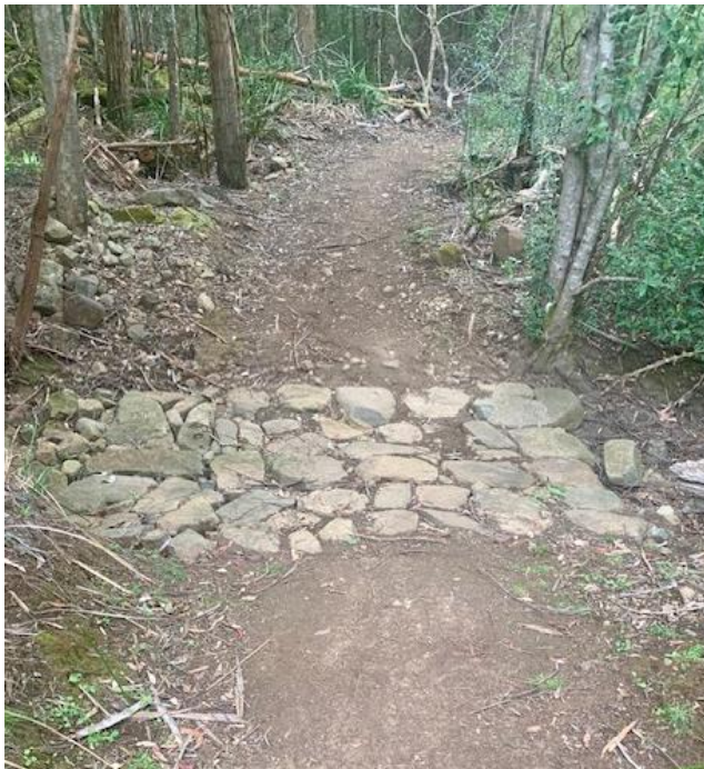
Images above showing rock armouring example from Stage 1
