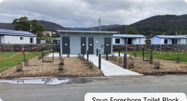
Snug Foreshore Toilet Block
