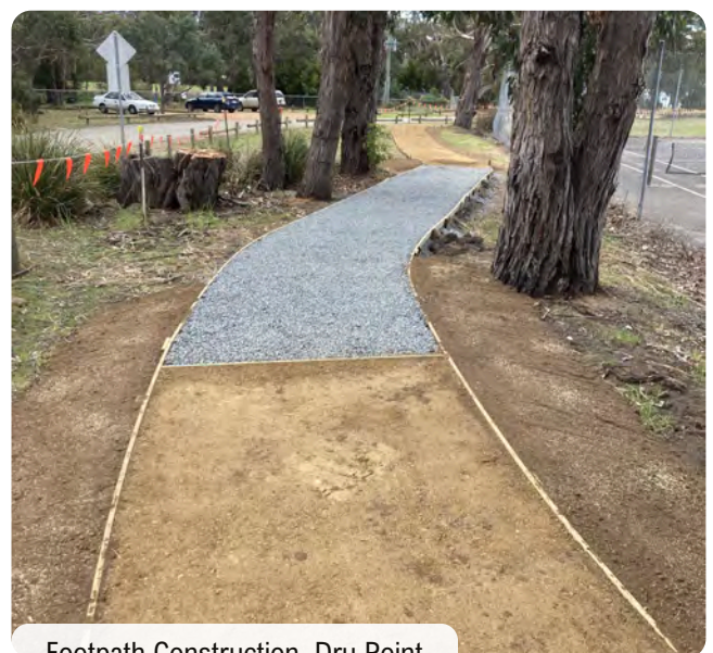
Footpath Construction, Dru Point
