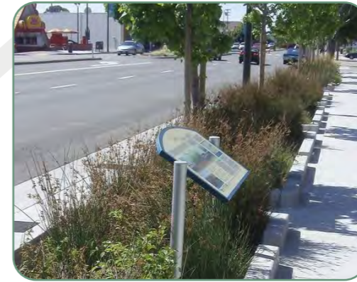
Areas for stormwater cleansing within on-street rain gardens.
