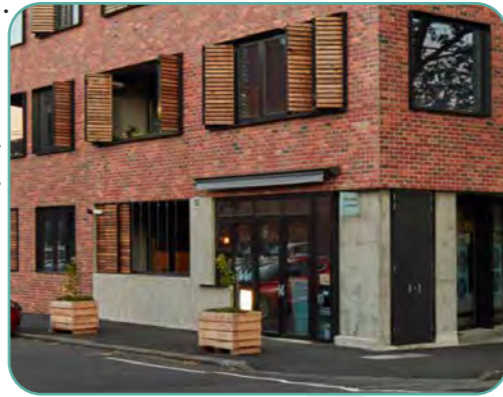
Ground floor commercial with residential uses above.
