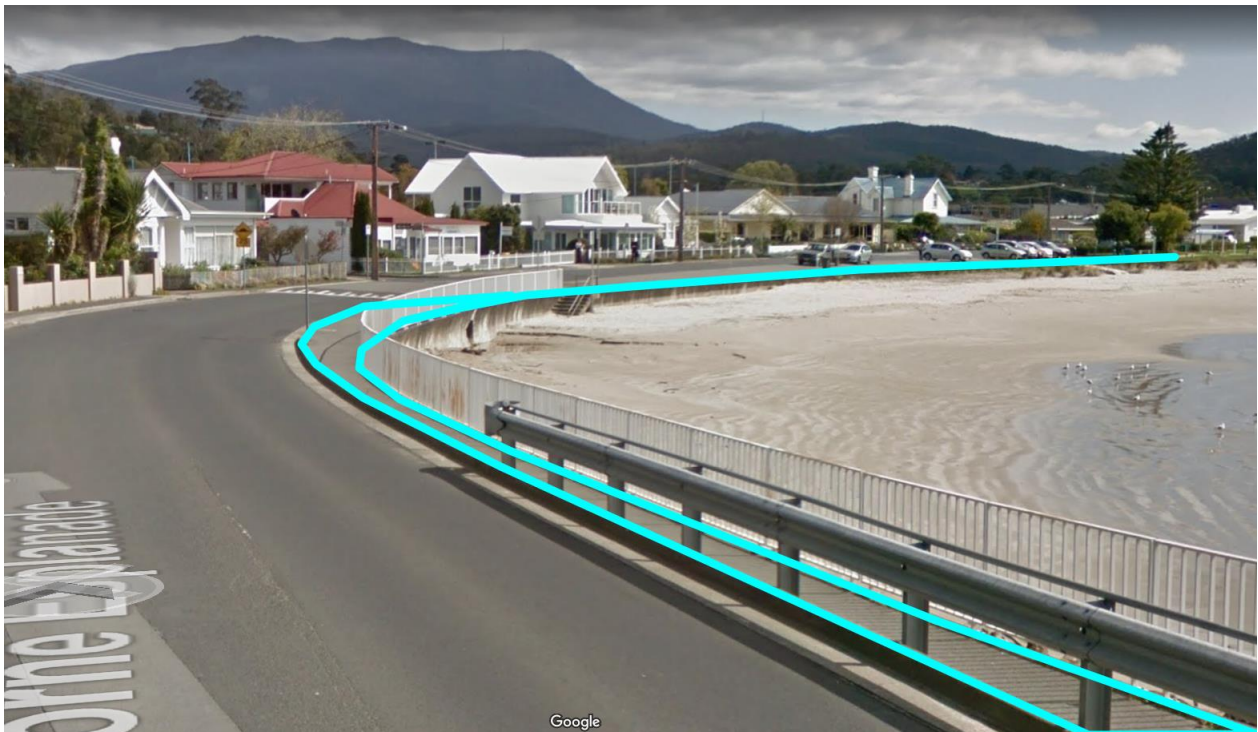
Photo 7: Proposed Sea Wall Upgrade – Raising the Footpath on Existing Sea Wall.
