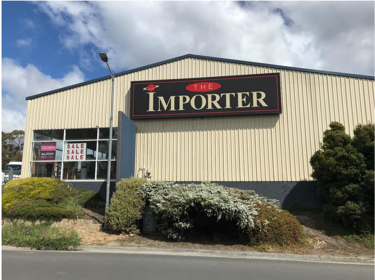
Figure 19: Image of the building showing the sign prior to its change to Total Tools.
