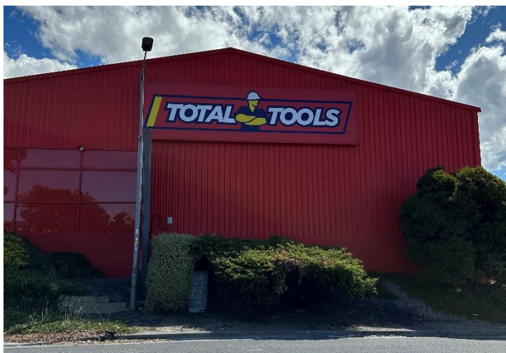
Figure 20: Image of the building showing the sign in its current form.
