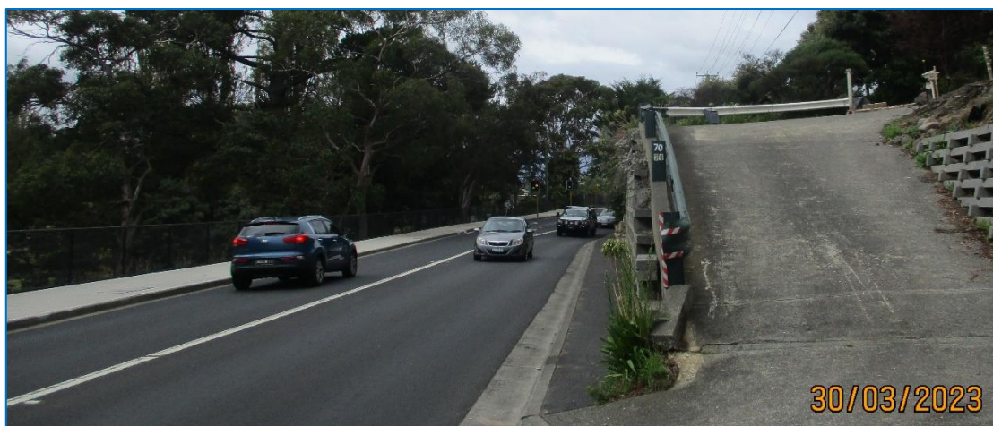
Photograph 7.2B – Available sight distance to the right (80 metres)
