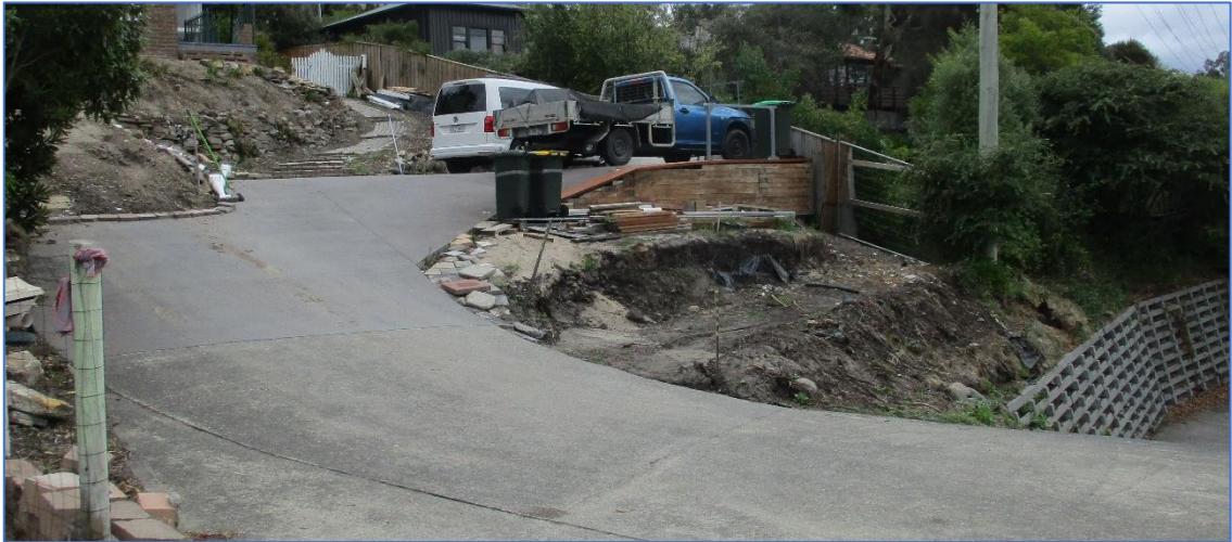
Photograph 5.4 – Access to property 74 (view from shared driveway)
