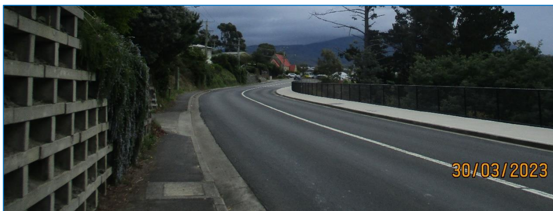
Photograph 7.2B – Available sight distance to the right (80 metres)
