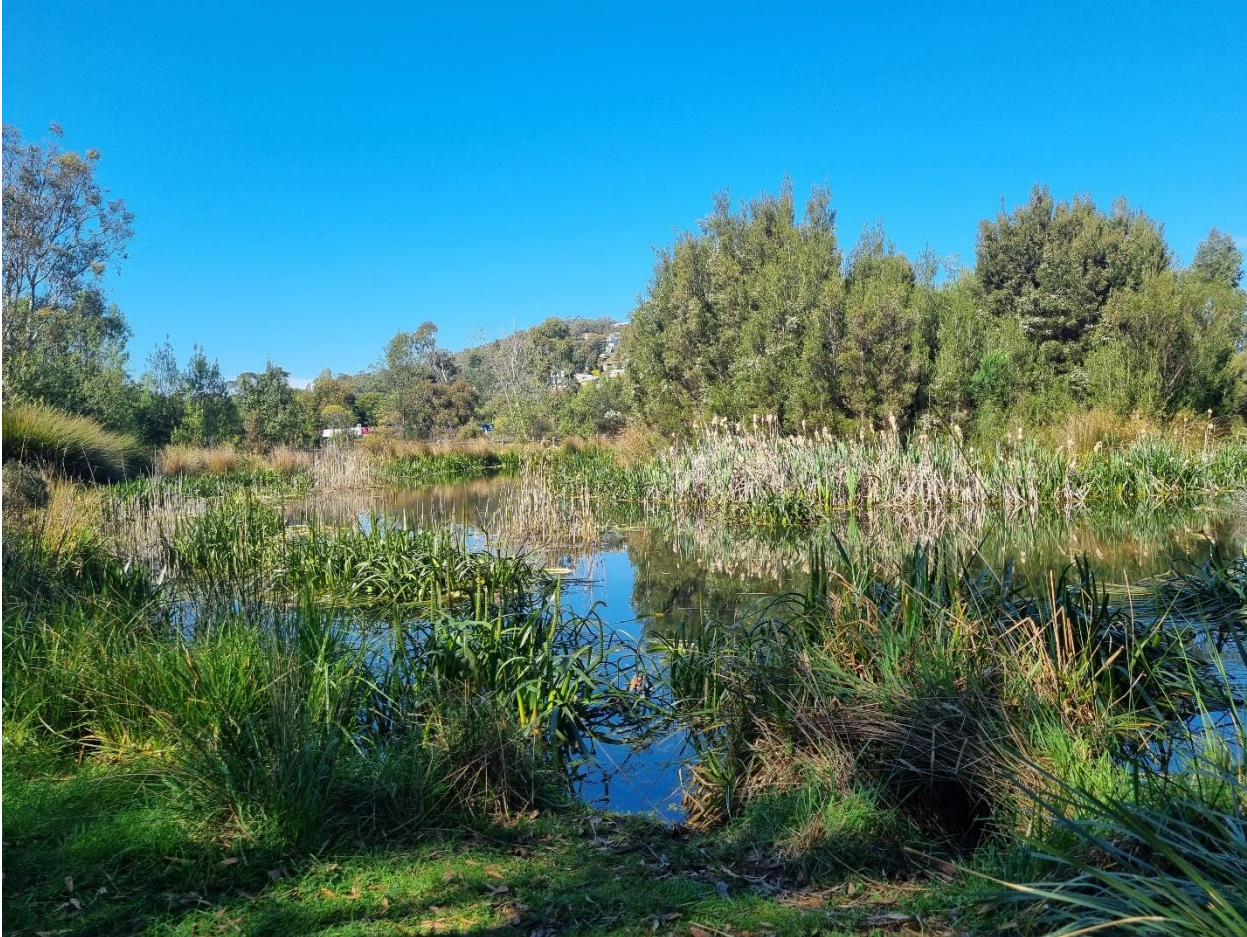
Photos of the Kingston Stormwater Wetlands
