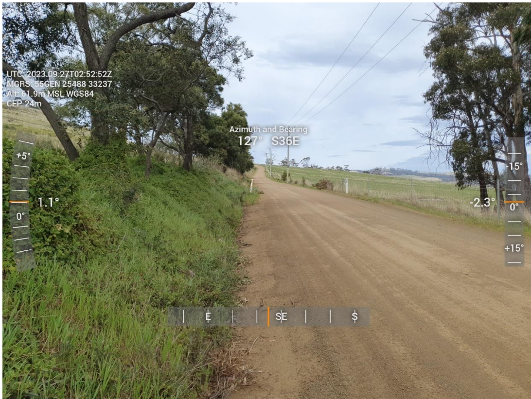
Figure 3.9 Tinderbox Road looking south-east from proposed balance lot access point frontage
