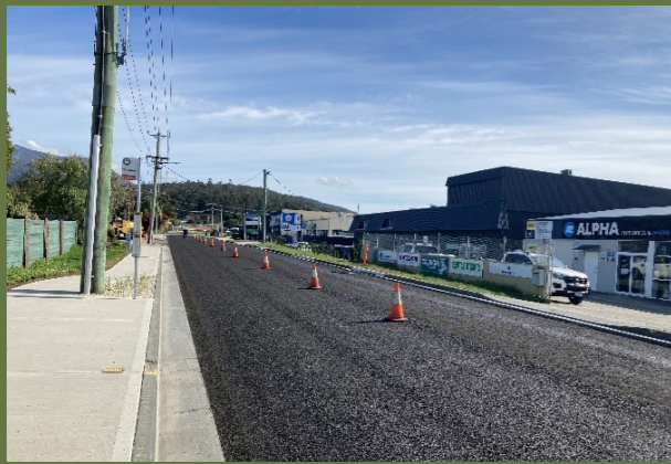
Reconstruction of Browns Road, Kingston - Stage 1
