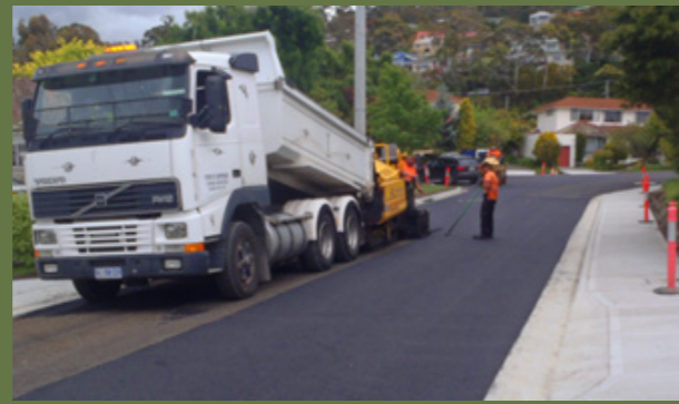
Completion of stormwater upgrades and road reconstruction of Meath Avenue, Taroom
