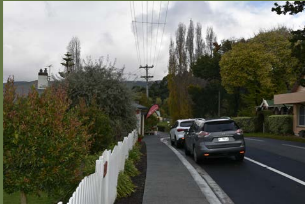
Construction of new sealed footpath on Channel Highway, Woodbridge
