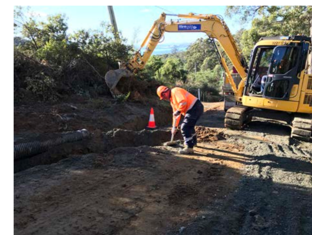
Work on Snug Tiers Road
