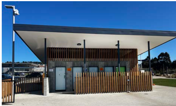
Newly constructed toilet block at Kingston Park
