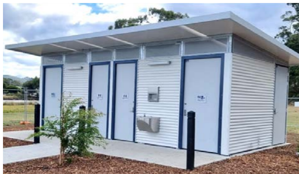
New toilet facilities constructed at the Christopher Johnson Reserve, Kingston
