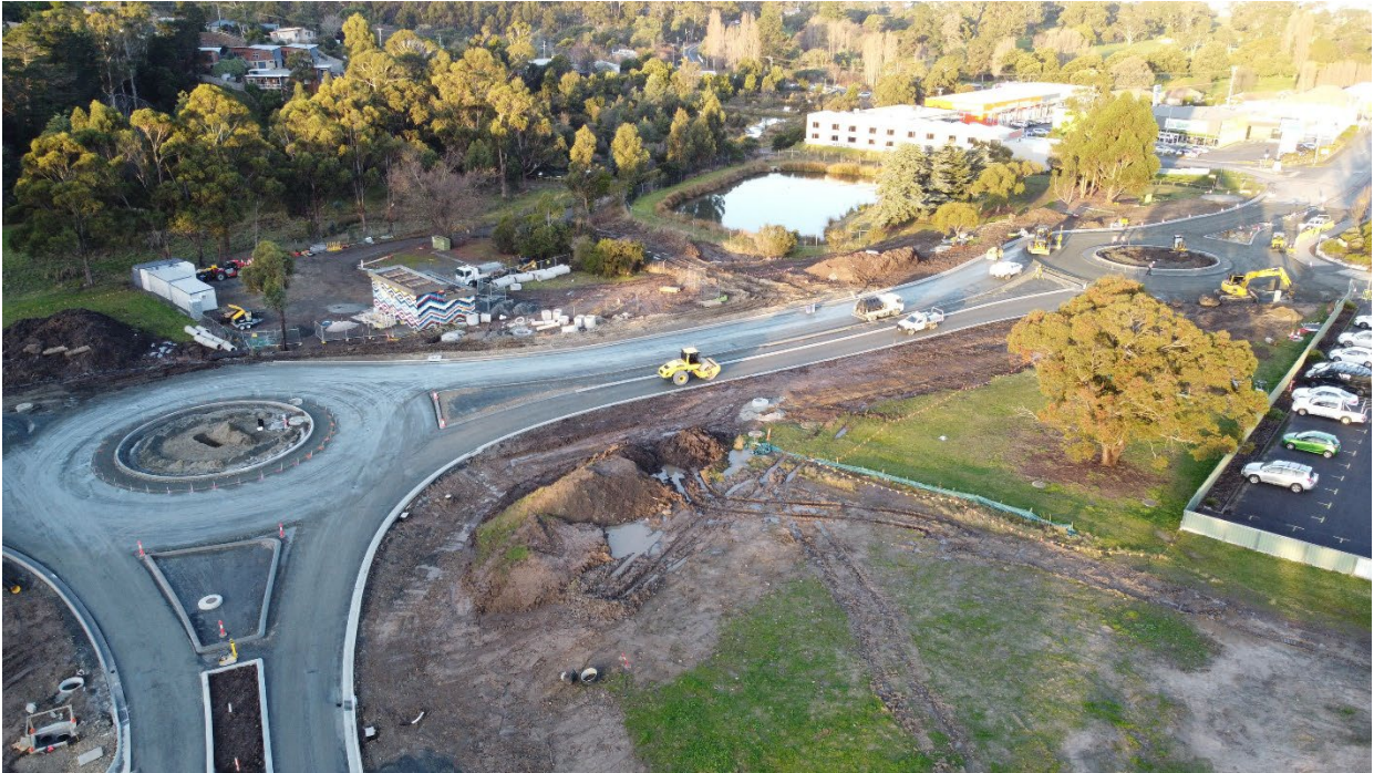
Figure 6 – Site progress as of 21 July
