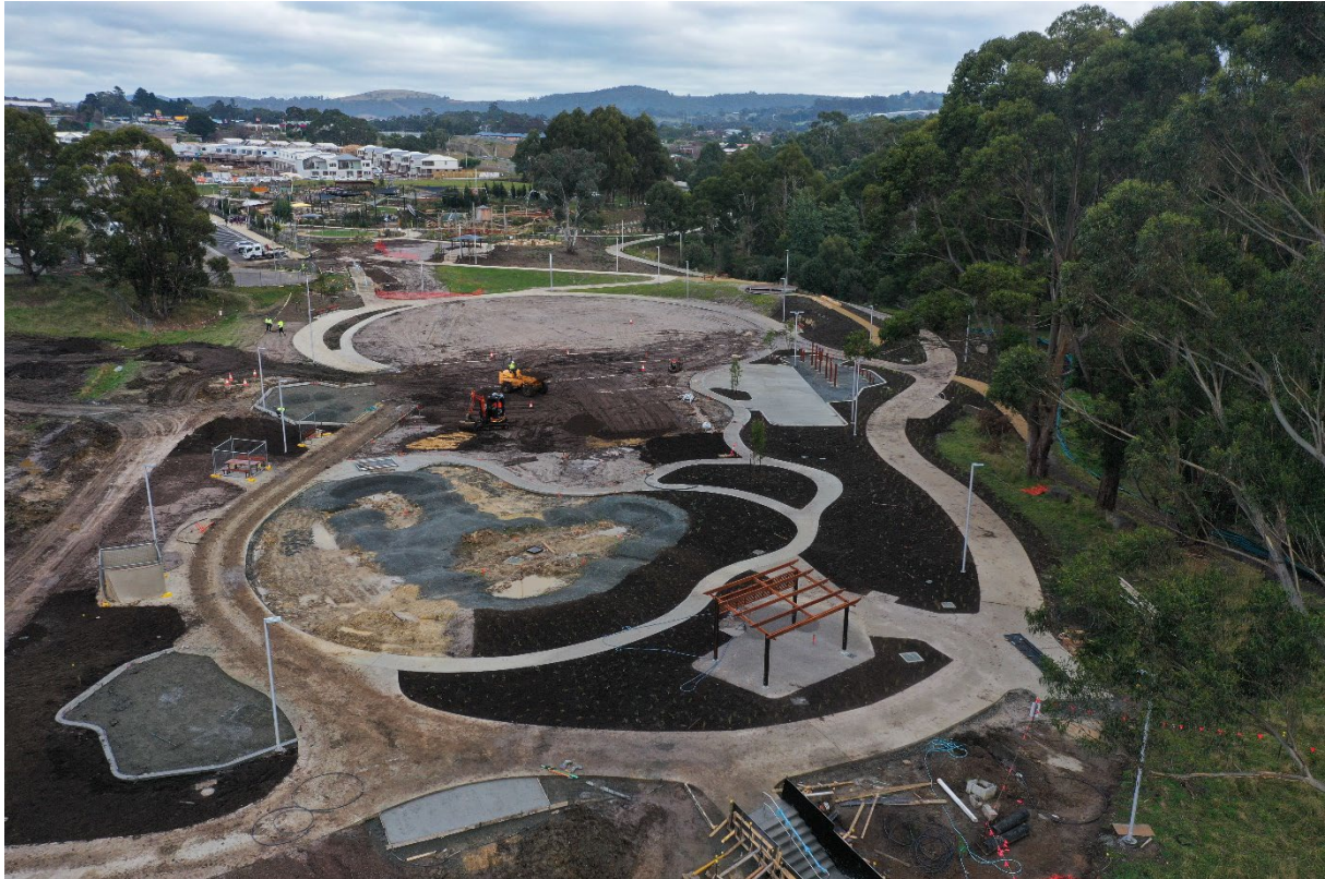
Figures 12a & 12b – site progress on P.O.S stage 2 as at July 2022
