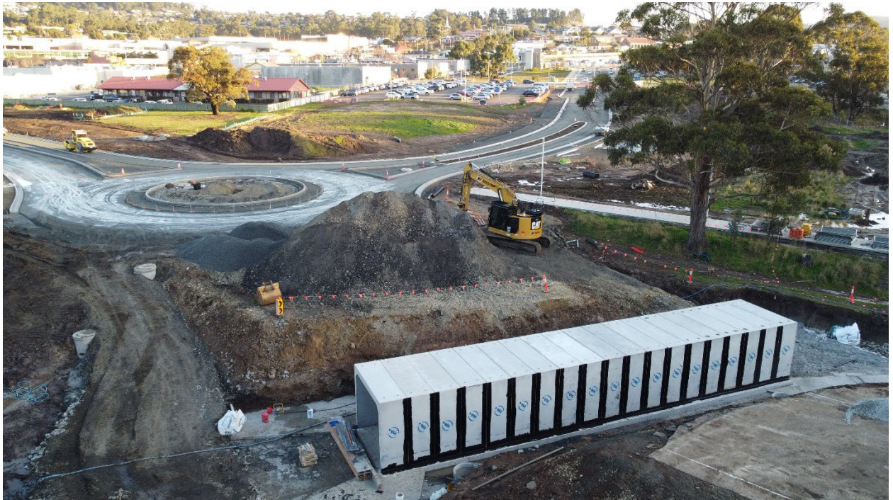
Figure 5 – Site progress as of 21 July
