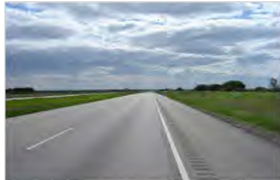
Figure 1 Sealed road shoulder
