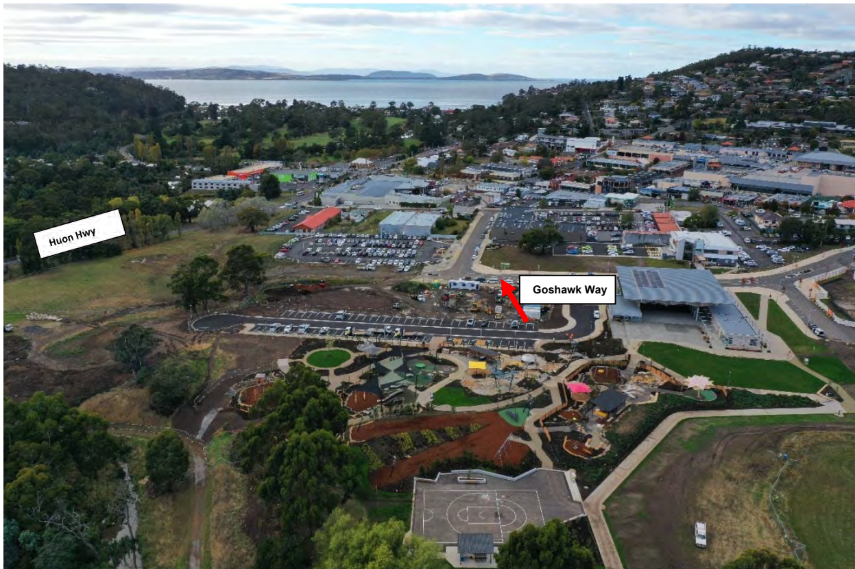
Figure 5 – Site in February 2020 (Goshawk Way will connect to Huon Highway)
