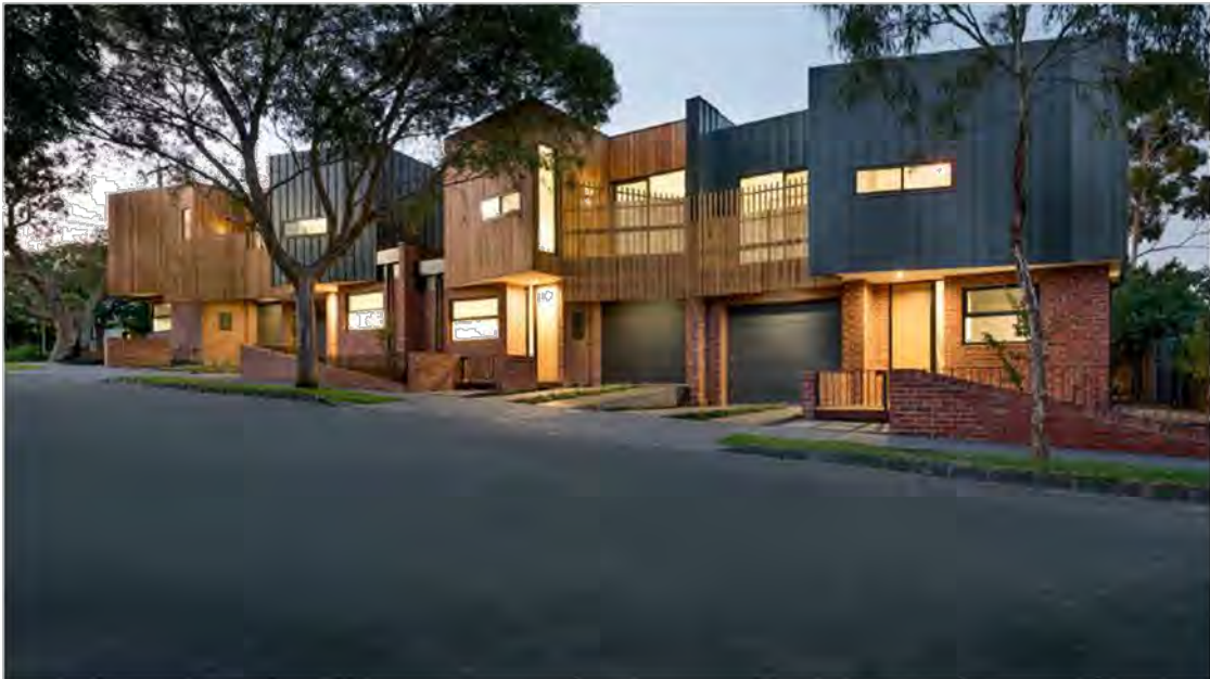
A simple materials palette. Alternating timber and metal cladding differentiates dwellings with consistent masonry podium.
