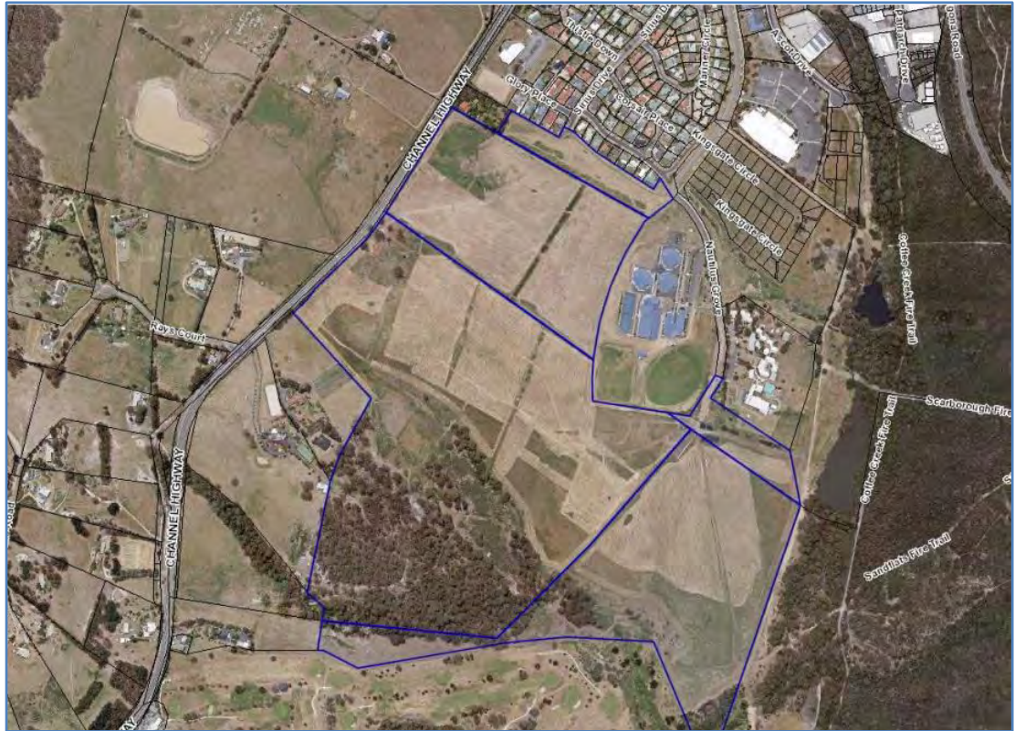
Figure 4 - Aerial photo of Huntingfield Land Supply Order land and area.
