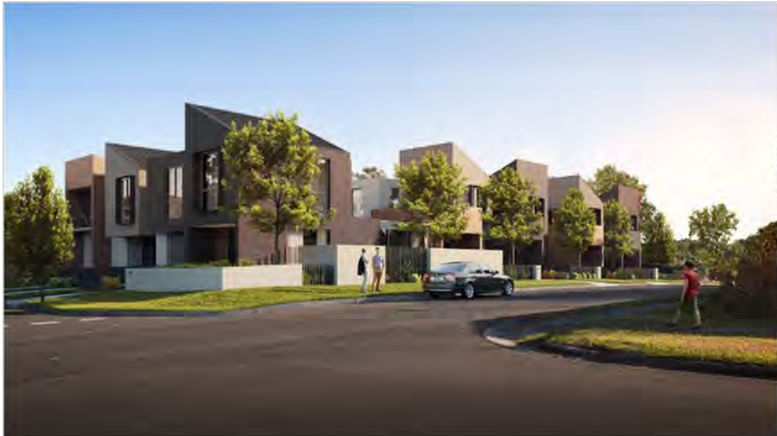
Articulated and varied building forms add visual interest. Trees enhance street and soften visual impact of dwellings.
