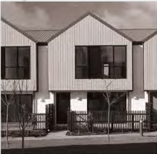
A good example of narrow terrace housing.
