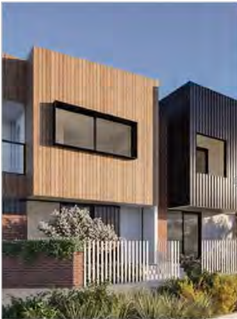
Good composition of timber elements with window openings, projecting beyond a masonry wall.
