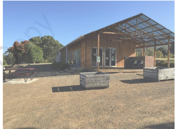
Figure 3: Lily Poulett-Harris Pavilion (north elevation), showing interface with driveway
